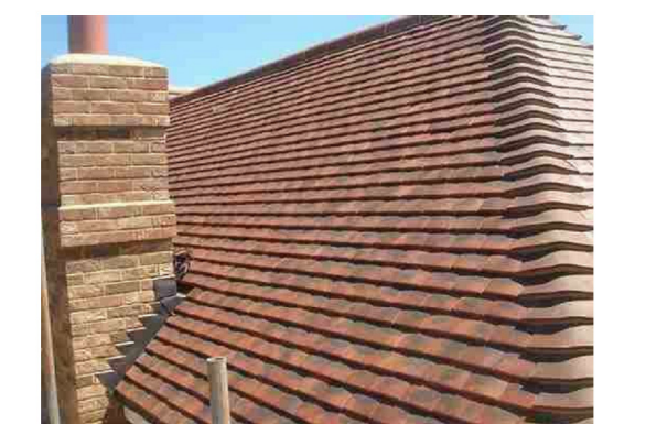
3. Handmade sandfaced plain tiles with bonnet tiles to hips
